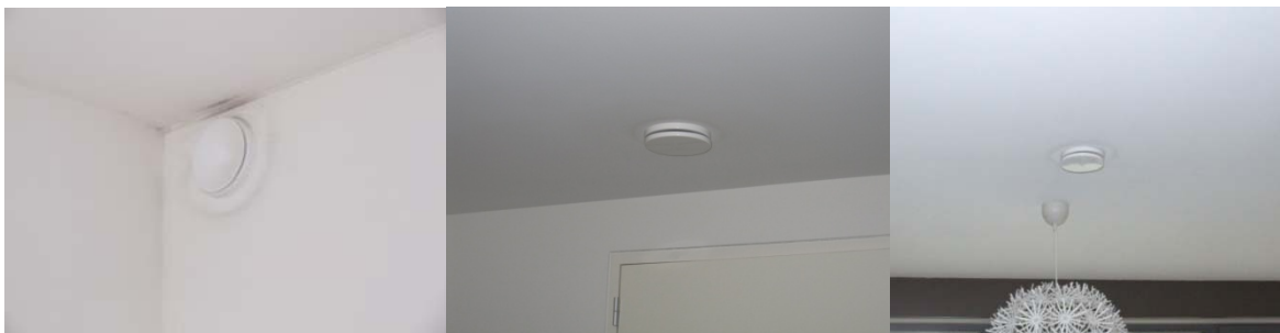
Figure 8 Examples of different (acoustically relevant) positioning of air inlets (MMP, MP and P)
